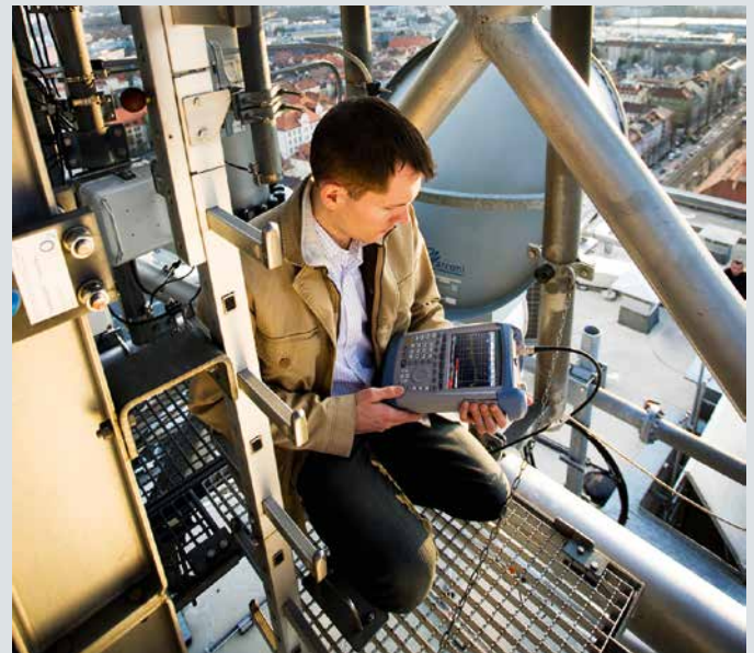
Fig. 2: Cost-efficient mobile T&M equipment is used to install a base station.
